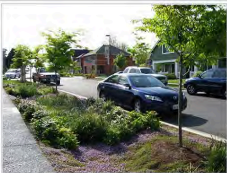
Street-side swale and adjacent pervious concrete sidewalk in Seattle , US. Stormwater is infiltrated through these features into soil, thereby reducing levels of urban runoff to city storm sewers .
